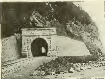
UTO TUNNEL, NIPPON RY., JAPAN.
